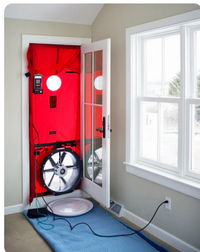
Figure 2: Blower door test
